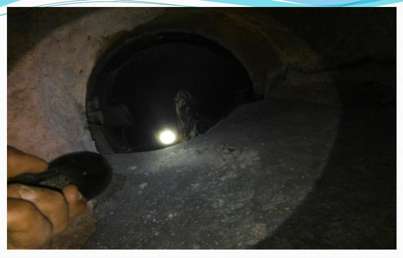
Catalyst heap upstream of MOV restricting its operation
