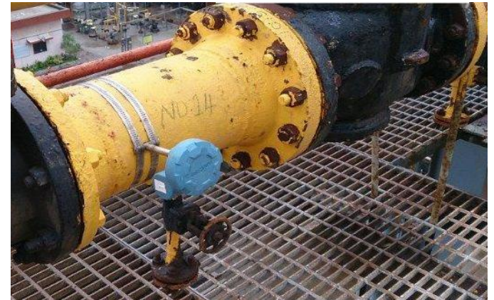
Wireless Acoustic transmitter installed on PRV
